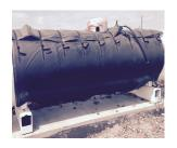
A large US railroad company uses these heaters to keep snow off the tracks. By applying Powerblanket Gas Cylinder Warmers to their 1000 lb propane tanks, they power their generators along the railway system. Before using the Powerblanket heaters, the cold temperatures kept the propane from vaporizing, which made it more difficult to remove snow becuase the generators did not work.
