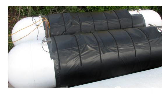
cold weather and molecular density. When temperatures drop, so does the pressure a fluid or gas can maintain, as the molecules move closer together. Keeping a tank at a temperature that will maintain the proper pressure may seem next to impossible. especially since most propane is stored outside even during the winter months.
