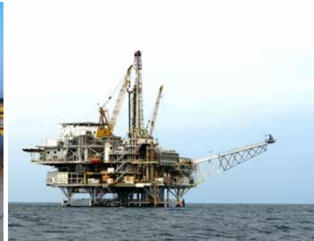
Solutions are tested before being commissioned
